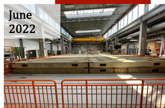
Completion of overburden installation
